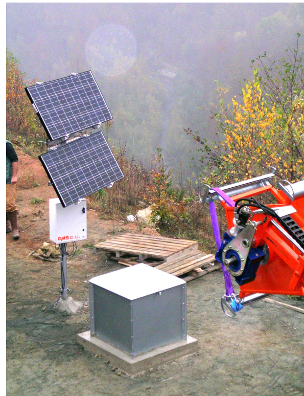
Figure 3 : DMS system installation completed
