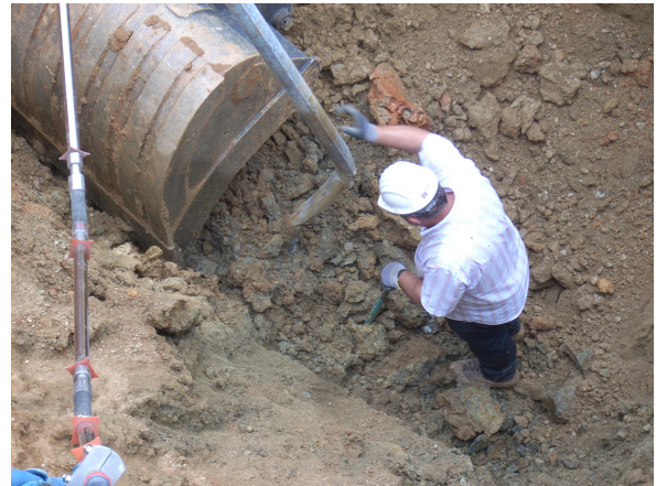
Figure 8 : Recovery of DMS column and displacement control
